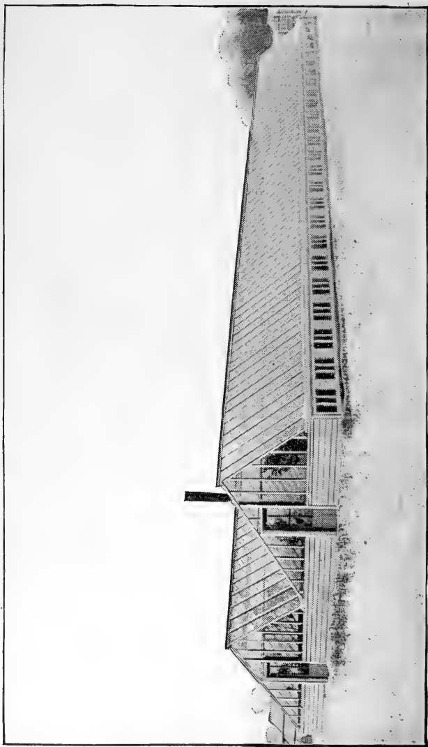
FIG. 36. SHORT SPAN TO THE SOUTH CARNATION HOUSES. ( Fred Dornier and Son, Lafayette, Ind. )
