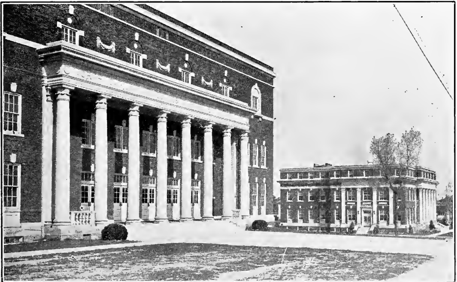
VIEW OF AYCOCK AUDITORIUM AND MUSIC BUILDING AT COLLEGE FOR WOMEN, UNIVERSITY OF NORTH CAROLINA
