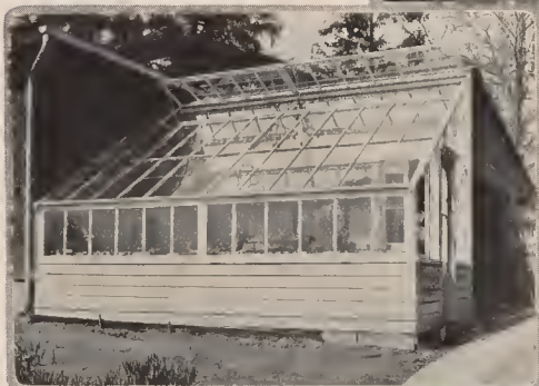
A simple type of lean-to greenhouse, showing the proper type of ventilator. For best results, the lean-to should be heated at night and on cold, cloudy days
