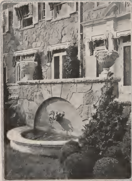
Ever since Moses struck the rock garden makers have built wall fountains. This is at the home of Earl P. Charlton, Westport Harbor, N. Y. Farley & Hooper were the architects
