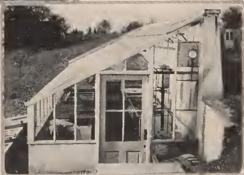
The lean-to above is built against a concrete wall. It is partly sunken and faces the south, to catch and hold the maximum amount of sun warmth
