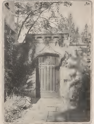
The garden gate of wide wooden planks can be elaborated with wrought iron strap hinges in character with the architectural design of the wall and the decorations upon it
