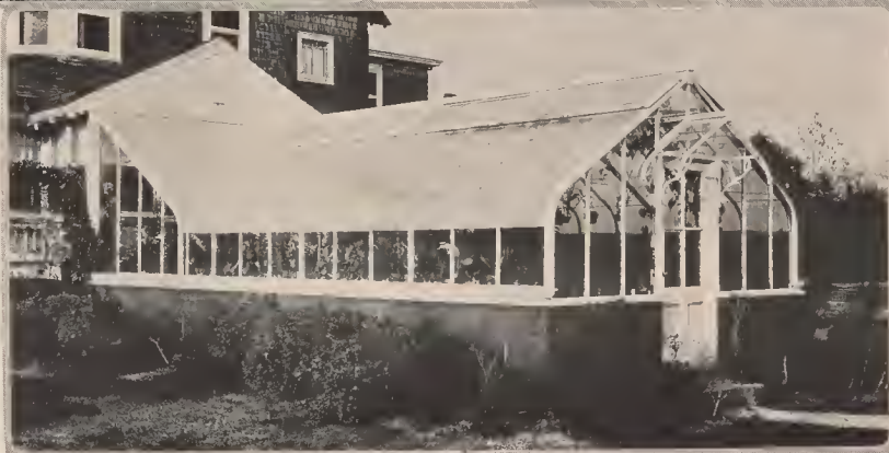
The lean-to above is built against a concrete wall. It is partly sunken and faces the south, to catch and hold the maximum amount of sun warmth
