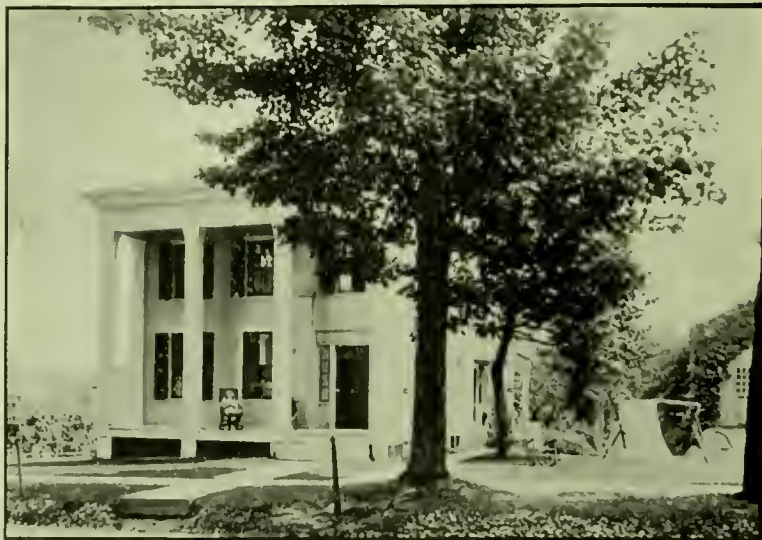
Dunwick, Photo. DR. CHARLES W. RADWAY'S RESIDENCE.
