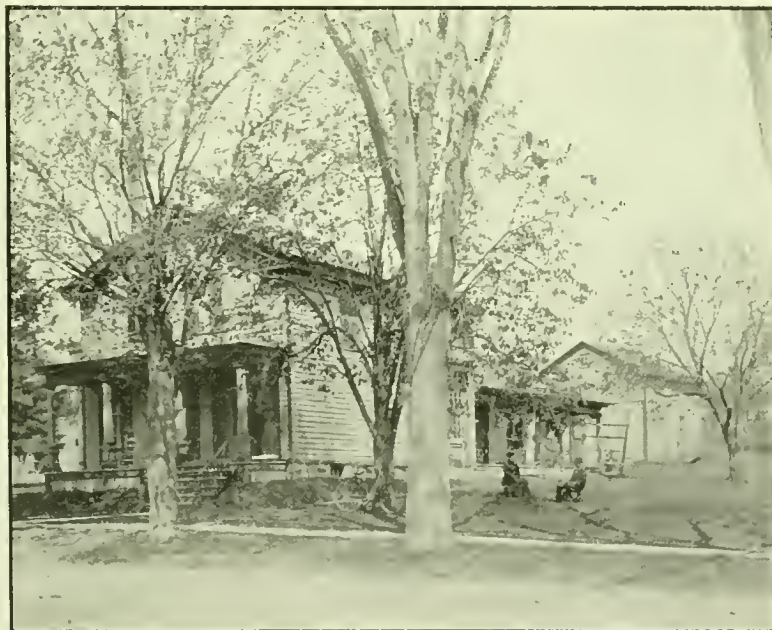
Borrowed Photo. HENRY HUMPHREY'S RESIDENCE.
