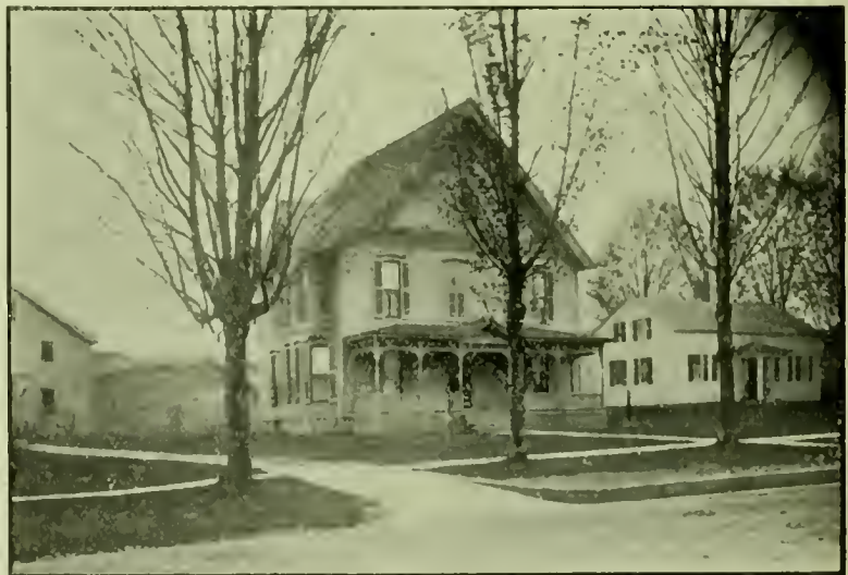
Dunwick, Photo. W. W. RINGSLEY'S RESIDENCE.
