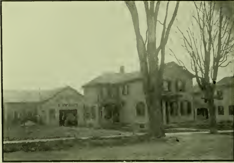
Dunwick, Photo. R. H. GREEN'S RESIDENCE AND LIVERY.
