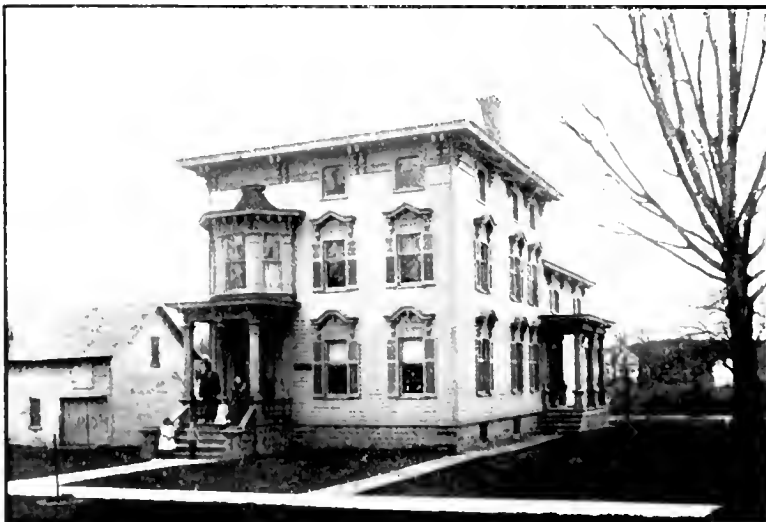
Dunwick, Photo. DR. E. S. SAMPSON'S RESIDENCE.
