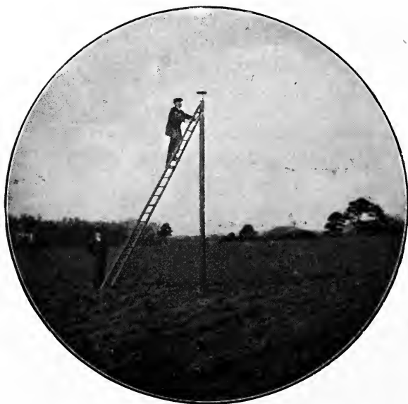
Placing an insulator upon one of the poles to carry electric discharge wire. The pole is fifteen feet high and the top portion of the insulator is about ten inches in diameter.
