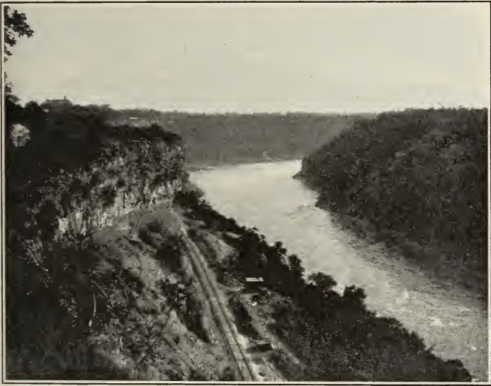
The Old or Lower Narrow gorge, looking south (up stream) from a point a little south of the mouth of the gorge near Lewiston. Track of New York Central railway in middle foreground. Lower end of Lower Great gorge at bend in distance. Niagara University at top on left. Water moderately turbulent, not placid as in Upper Great gorge or Lower Great gorge above Foster rapids.
