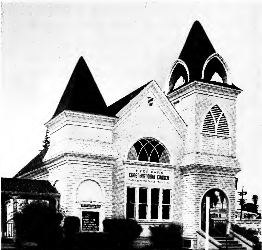
I 2,1. Hyde Park Congregational Church. Chatsworth, San Fernando Valley. 1901 (photo: Cultural Heritage Board, City of Los Angeles)
