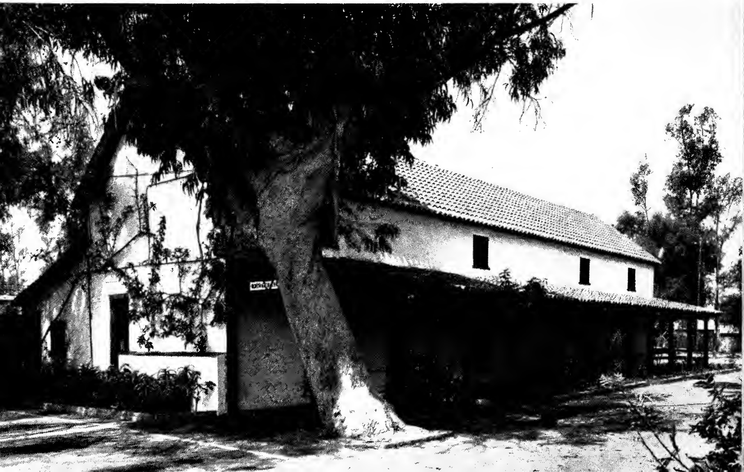
I 3,1. Andres Pico House. City of San Fernando. c. 1834 (photo: Cultural Heritage Board, City of Los Angeles)
