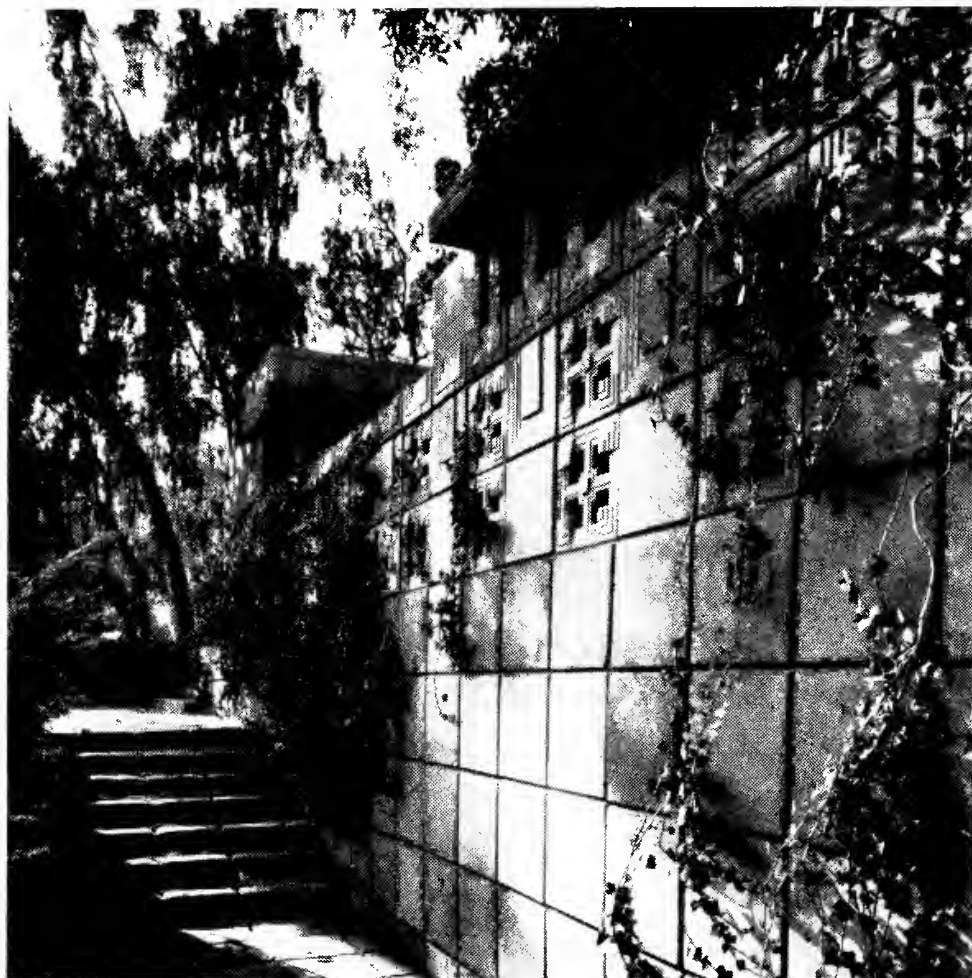
C 1,17. Storer House. Hollywood Hills. Los Angeles. 1923. Frank Lloyd Wright (photo: Julius Shulman)
