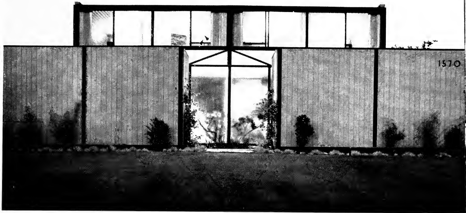
C 2,18. Courtyard Apartments. Hollywood, Los Angeles. 1952. Craig Ellwood (photo: Marvin Rand)
