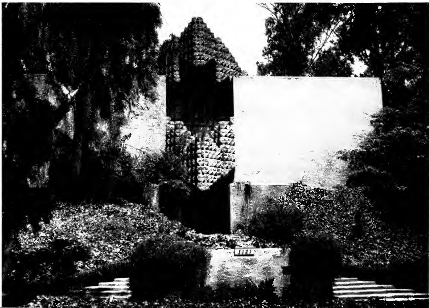
D 2,2. Sowden House. Griffith Park District, Los Angeles. 1926. Lloyd Wright (photo: authors)
