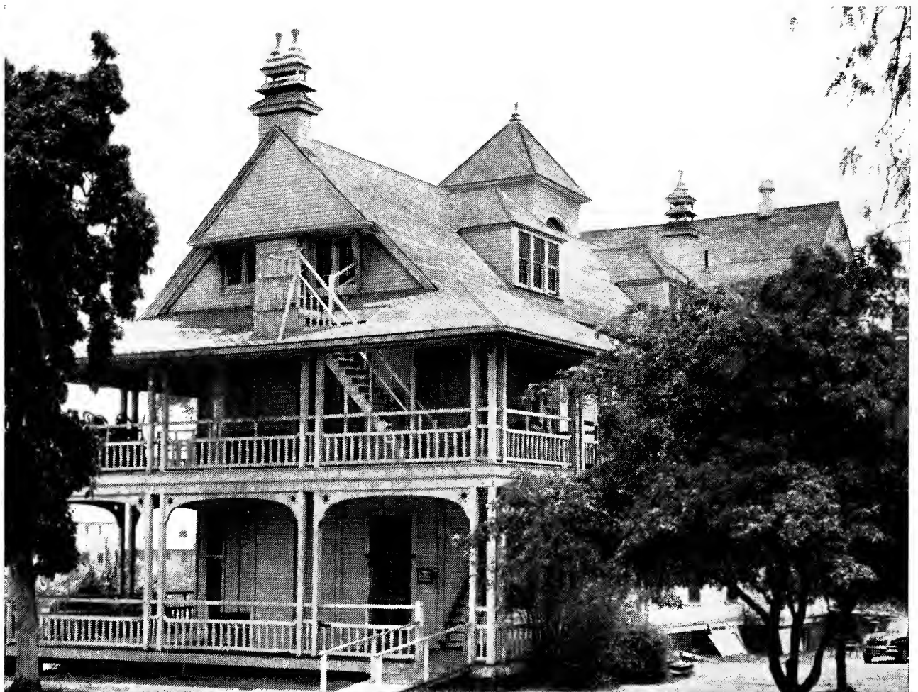
B 2,3. Sawtelle Veteran's Administration Center (Barracks). Los Angeles. 1901. Peters and Burns (photo: C. Winslow)
