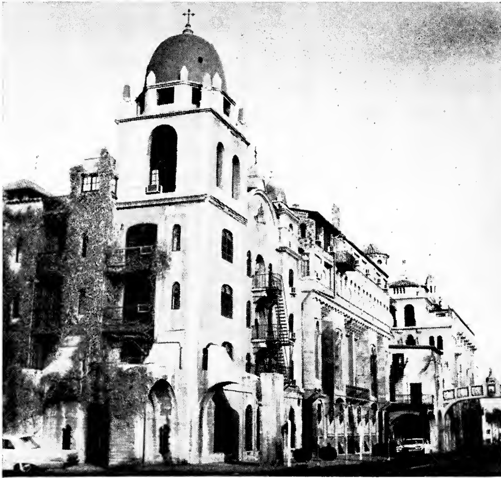
N 2,5. Mission Inn. Riverside. 1890—1901. Arthur Benton (photo: authors)
