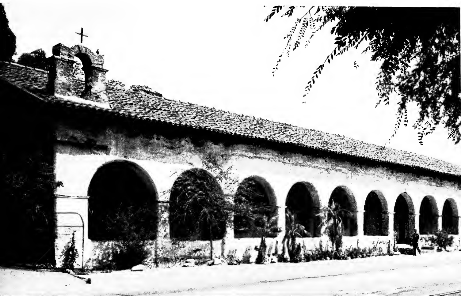
I 3,2. San Fernando Mission. City of San Fernando. 1818 (photo: Cultural Heritage Board, City of Los Angeles)
