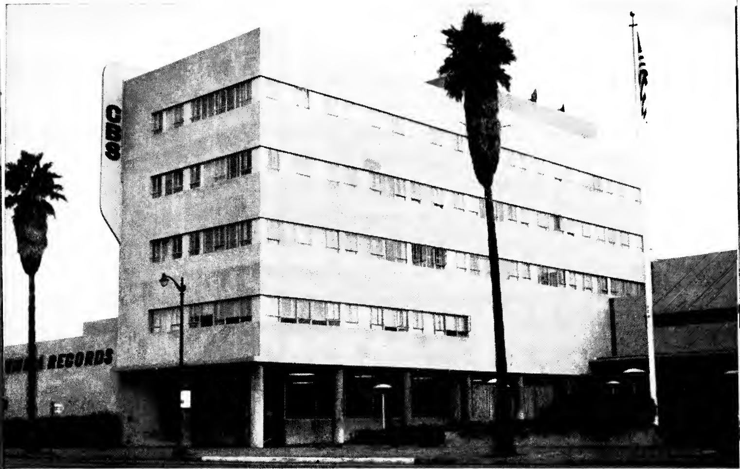
C 2,17. CBS Radio Building. Los Angeles. 1937–38. William Lescaze and E. T. Heitschmidt (photo: authors)
