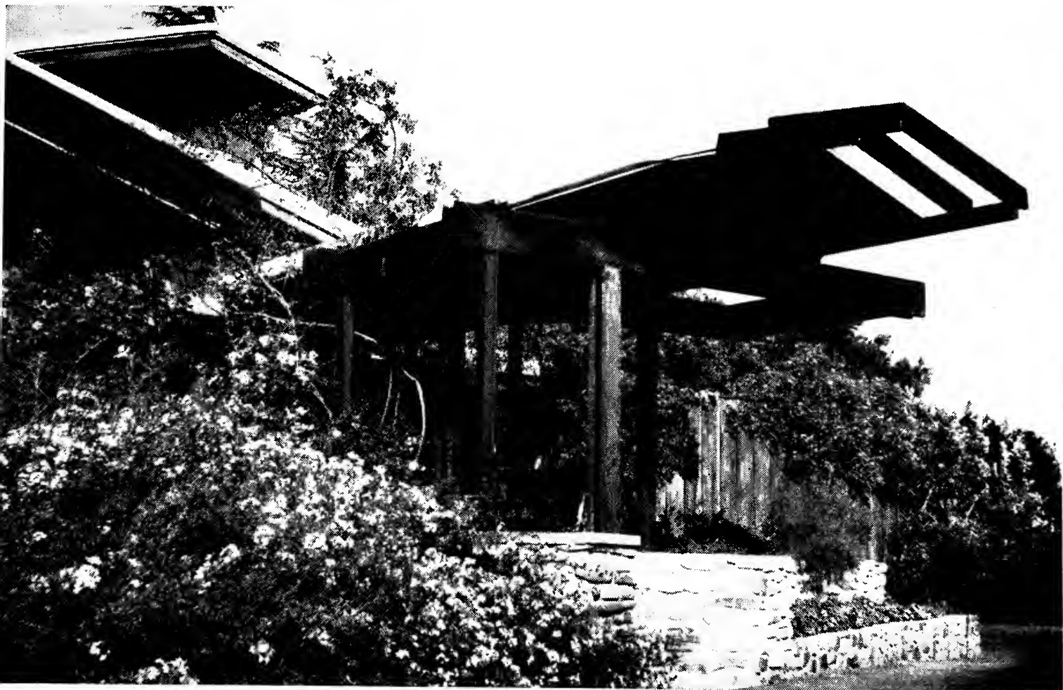
L 4,6. Wyle House. Ojai. 1947. Harwell Hamilton Harris (photo: authors)
