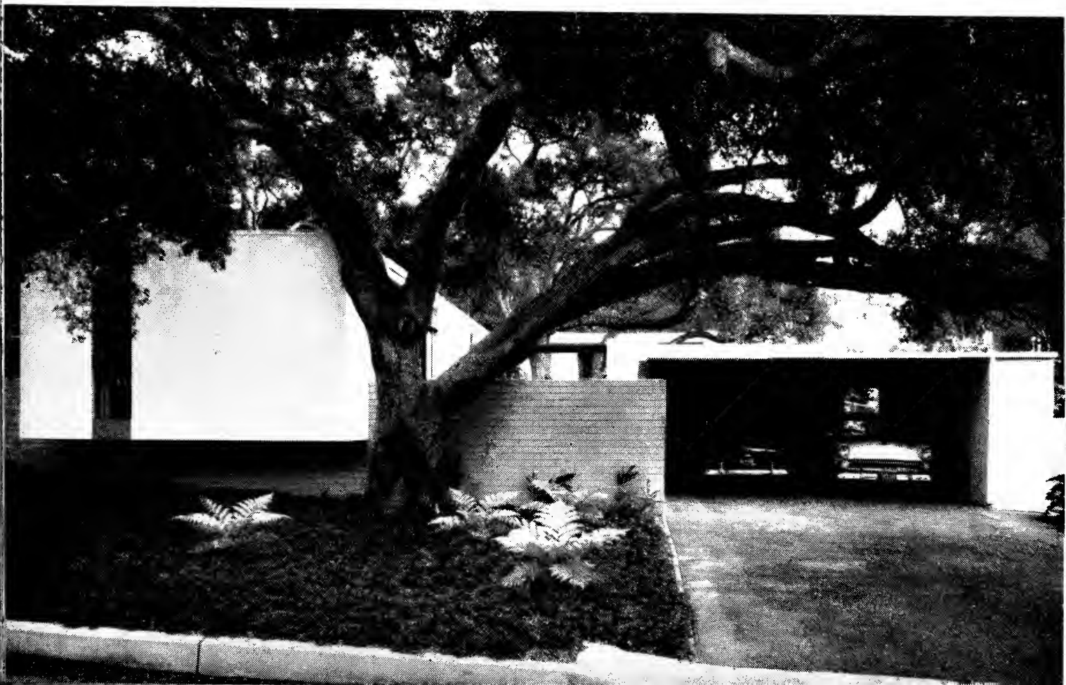
A 3,1. Emmons House. Pacific Palisades. 1954. A. Quincy Jones and Frederick E. Emmons (photo: Julius Shulman)
