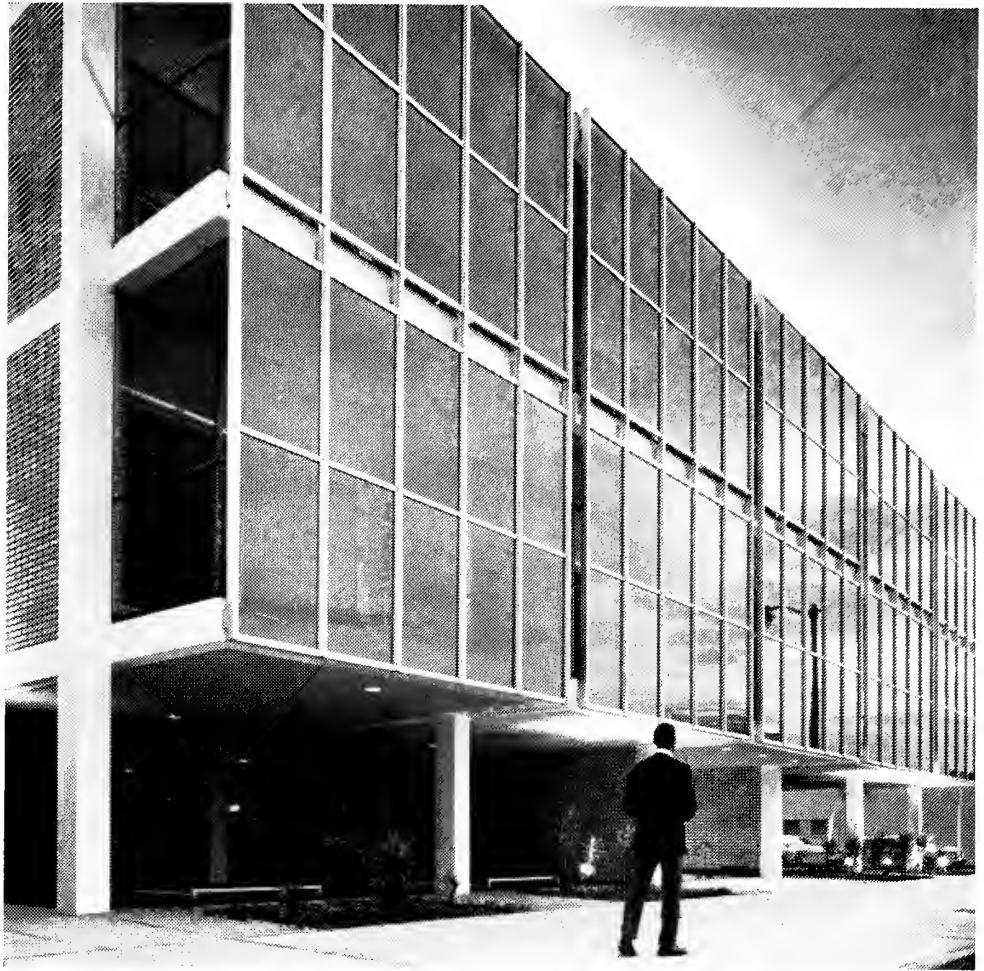
C 2,5. Carson-Roberts Building. Los Angeles. 1959. Craig Ellwood (photo: Marvin Rand)
