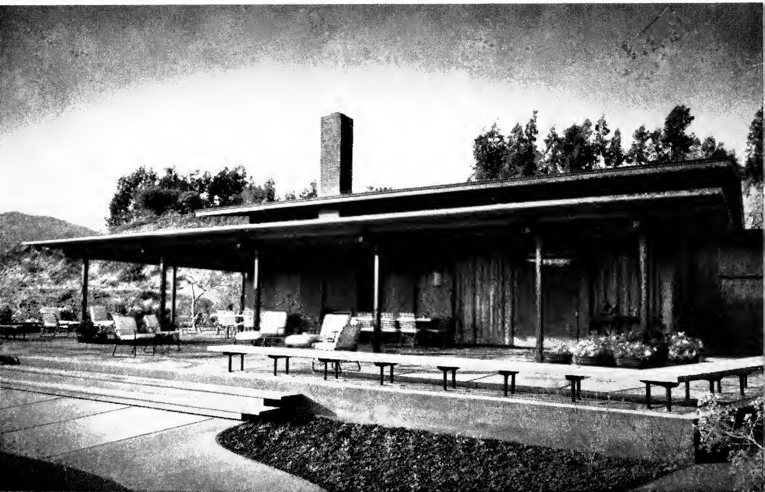
B 1,3. Sperry House. Brentwood Heights, Los Angeles. 1953. William Wurster, Bernardi and Emmons (photo: Julius Shulman)
