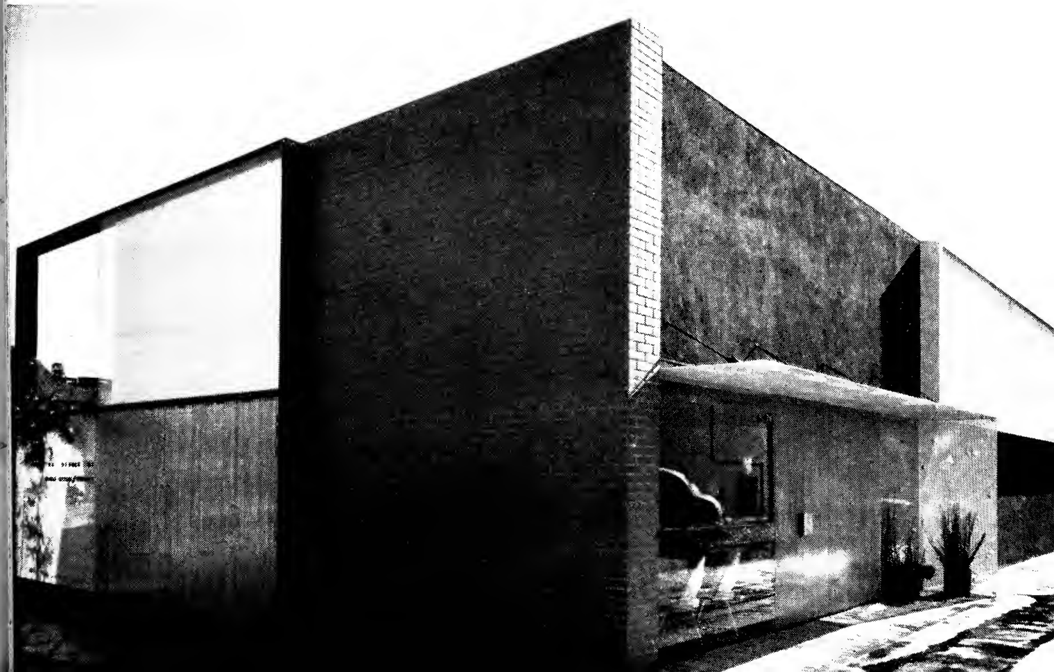
B 7,2. Beckett Office Building. Los Angeles. 1950. William S. Beckett (photo: Julius Shulman)
