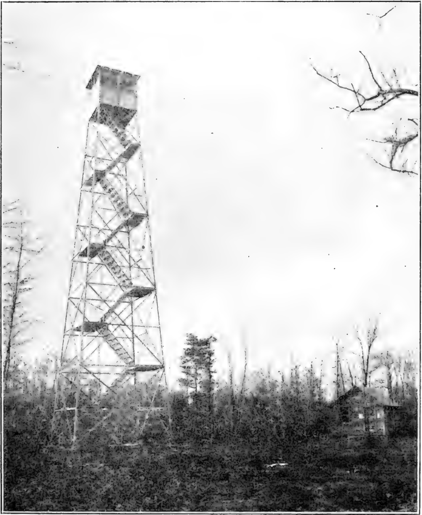
A MODERN STEEL FOREST FIRE TOWER. IT IS 60 FEET HIGH AND FROM ITS TOP MAY BE VIEWED 500,000 ACRES OF FOREST LAND.
