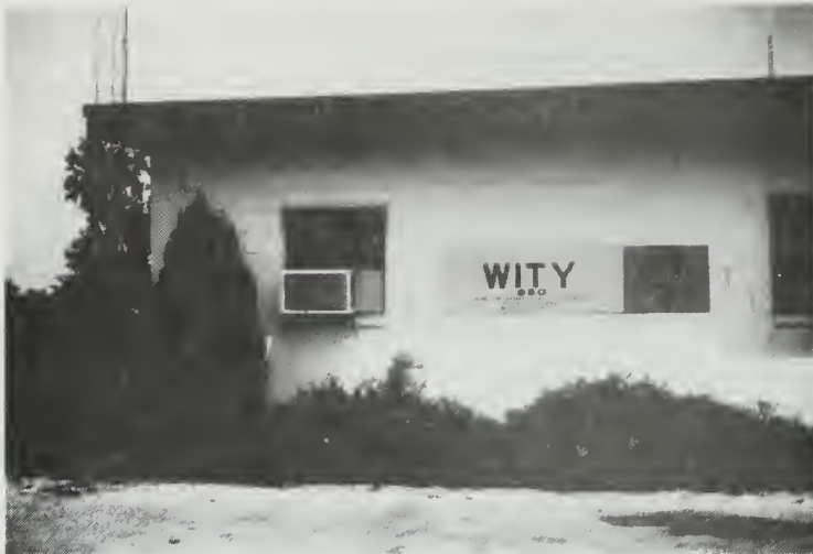
8b. Cracks that developed in concrete block wall. (DuMontelle, 1967.)
