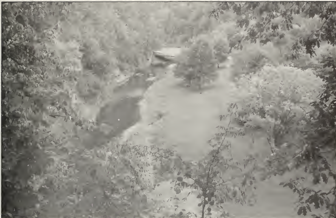
Figure 20 North Fork of Apple River at the Primrose Trail observation platform (photo by W. T. Frankie).
