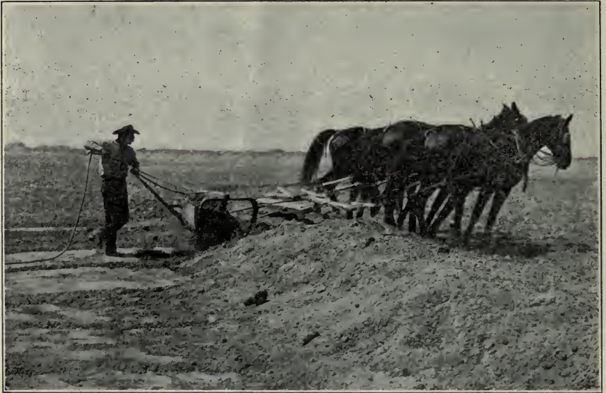
MAKING CHECK-LEVEE WITH FRESNO SCRAPER
