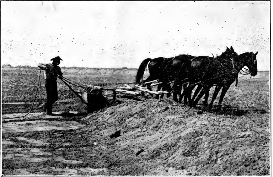
MAKING CHECK-LEVEE WITH FRESNO SCRAPER
