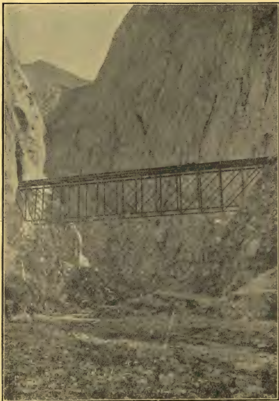
BRIDGE OVER THE HIGHEST R. R. IN THE WORLD—OROYA R. R.
