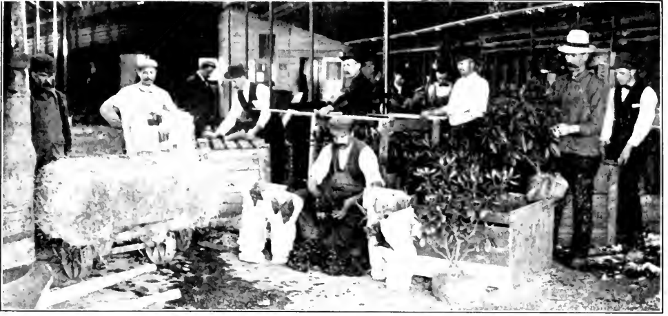
A CORNER IN ONE OF THE PACKING ROOMS.
