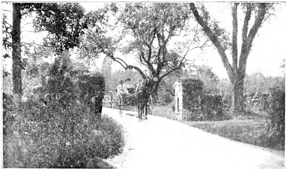
ENTRANCE GATE ON WESTOVER ROAD.
