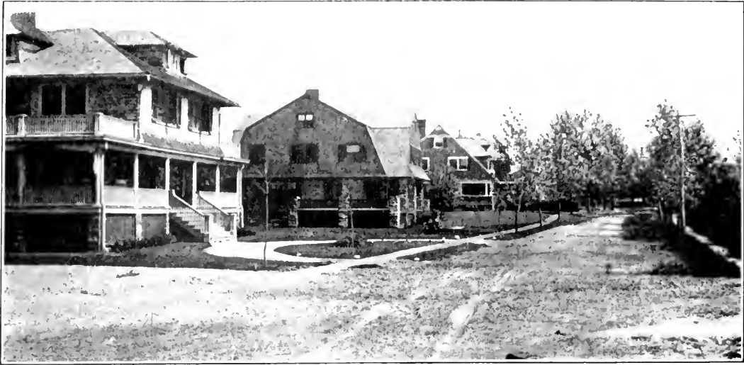
NAWTHORNE STREET, SHOWING ITS APPEARANCE SO FAR AS DEVELOPED. Looking eastward from the beach land.
