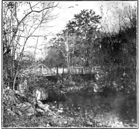
THE BRIDGE AT THE OLD WIRE MILLS.
