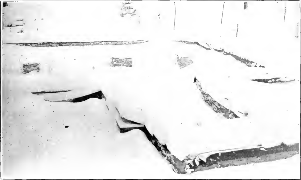
THE FOUNDATION COVERED WITH SNOW. Beautiful but not Efficient!
