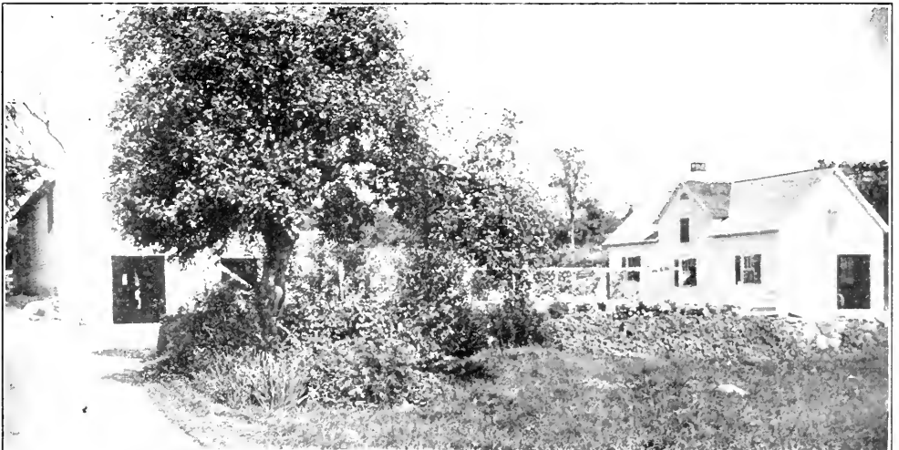
AN ATTRACTIVE APPROACH TO THE GARAGE.
