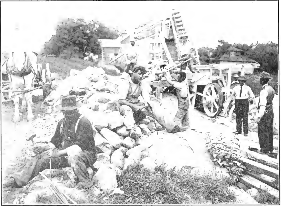
STAMFORD GRINDS UP ITS DISCARDED STONE WALLS.
