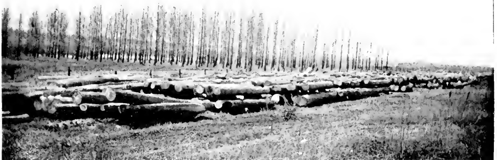
THE RIVER BANK IS LINED WITH LOGS.
