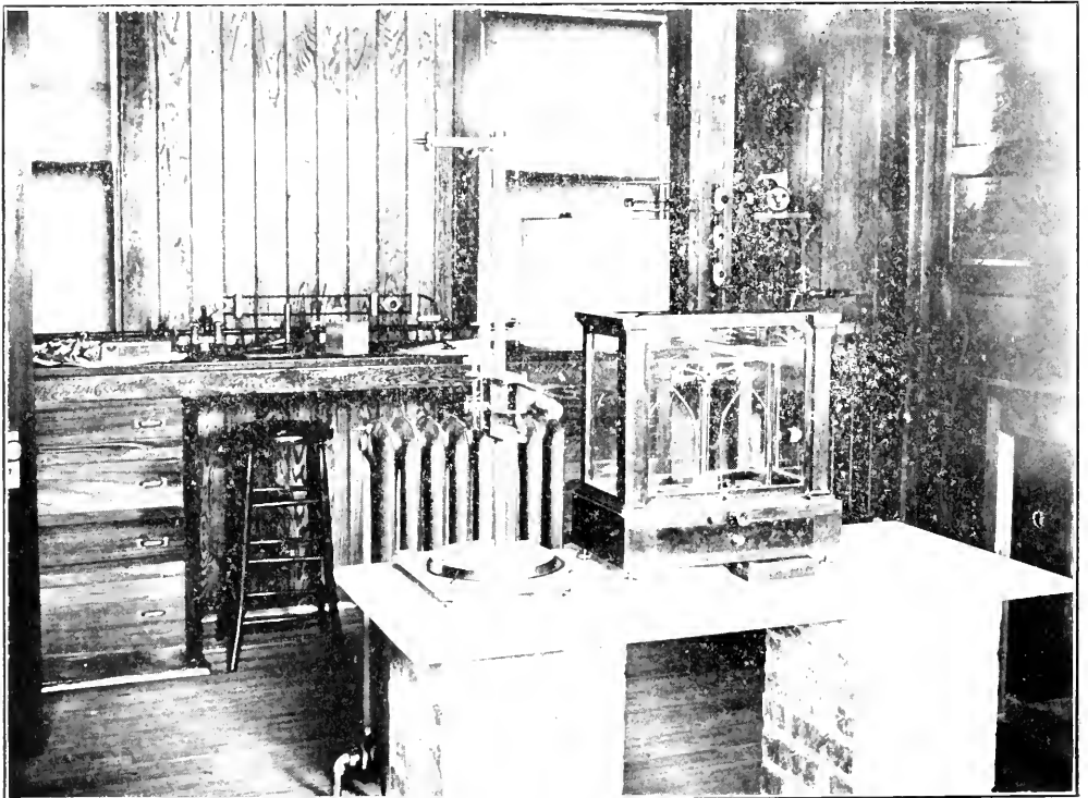
MAIN LABORATORY SHOWING VIBRATION-FREE SUPPORTS.
