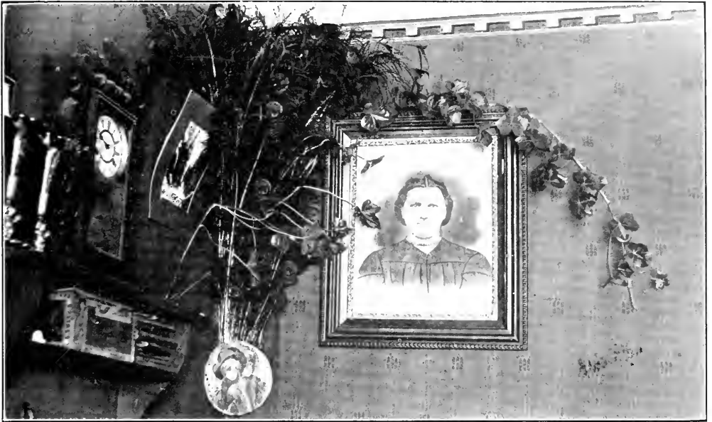
LIVING IVY THAT MADE ITS WAY THROUGH WALLS AND WALL PAPER.
