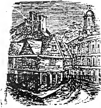
BUILDING FORMERLY CORNER K SQUARE AND ANN STREET (NOW NORTH).
