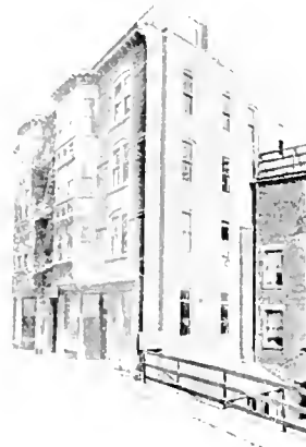
BUILDING LEWIS STREET EXTENSION. M. A. SLAVIN, BUILDER.
