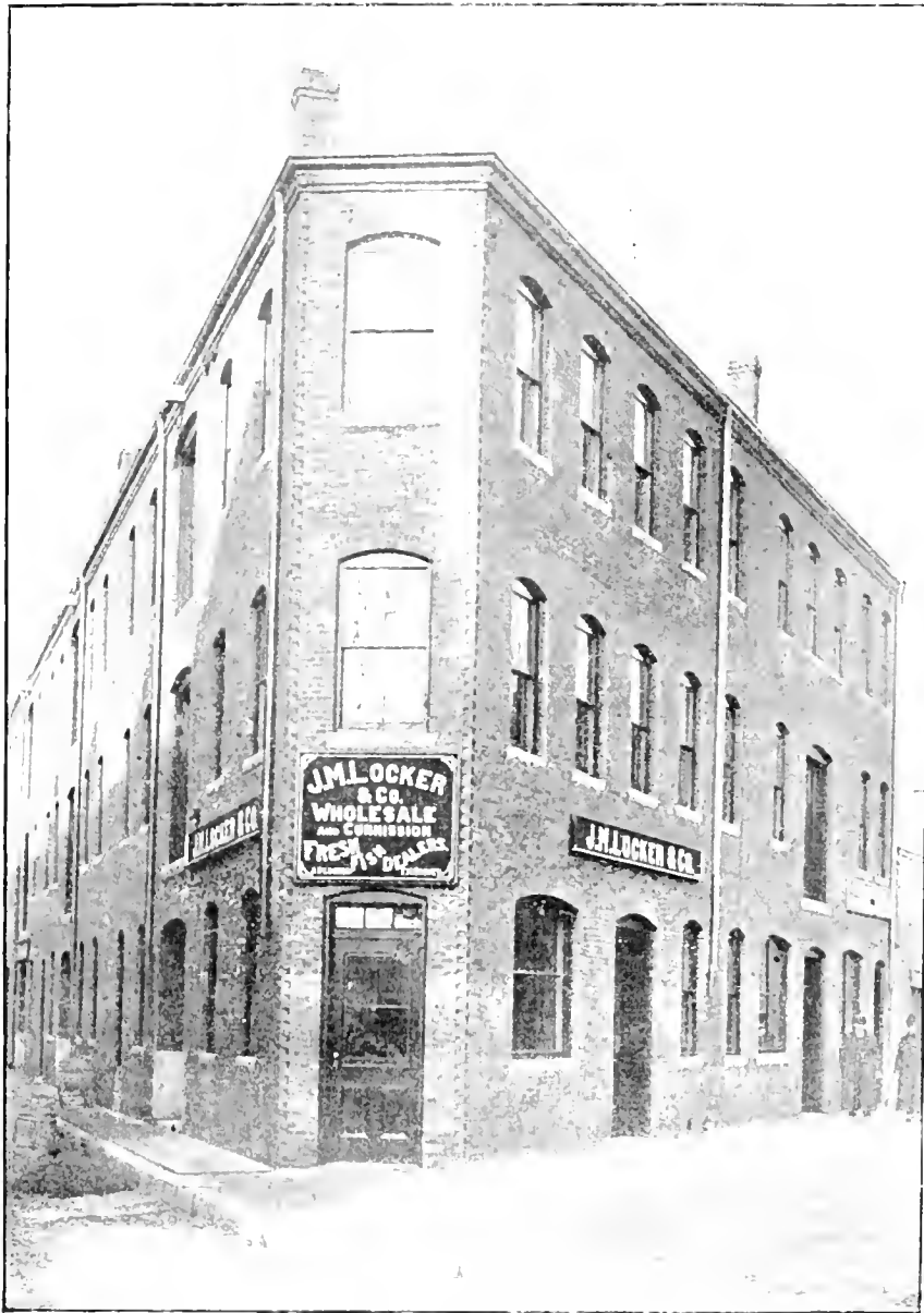
BUILDING, COMMERCIAL WHARF AND ATLANTIC AVENUE. BY PERMISSION OF M. F. SULLIVAN.
