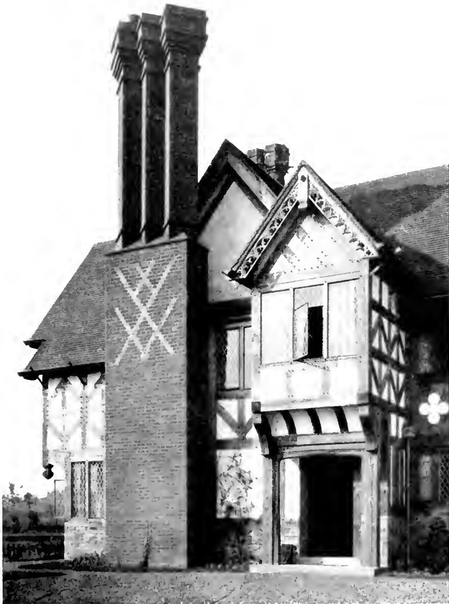
••The Gables," Thelwall, England, one of the comparatively few modern houses where the timbering is solid and extending the full depth of the wall
