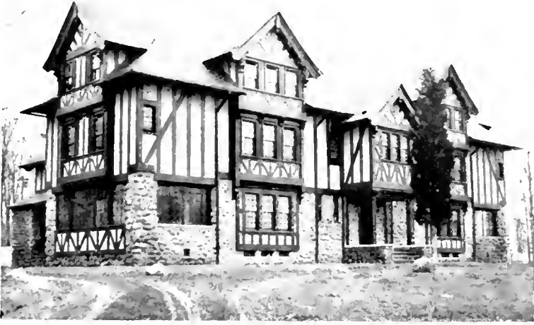
A modern half timber house at Essex Fells, N. J., with the typical diagonal end-braces and greater elaboration in the bays
