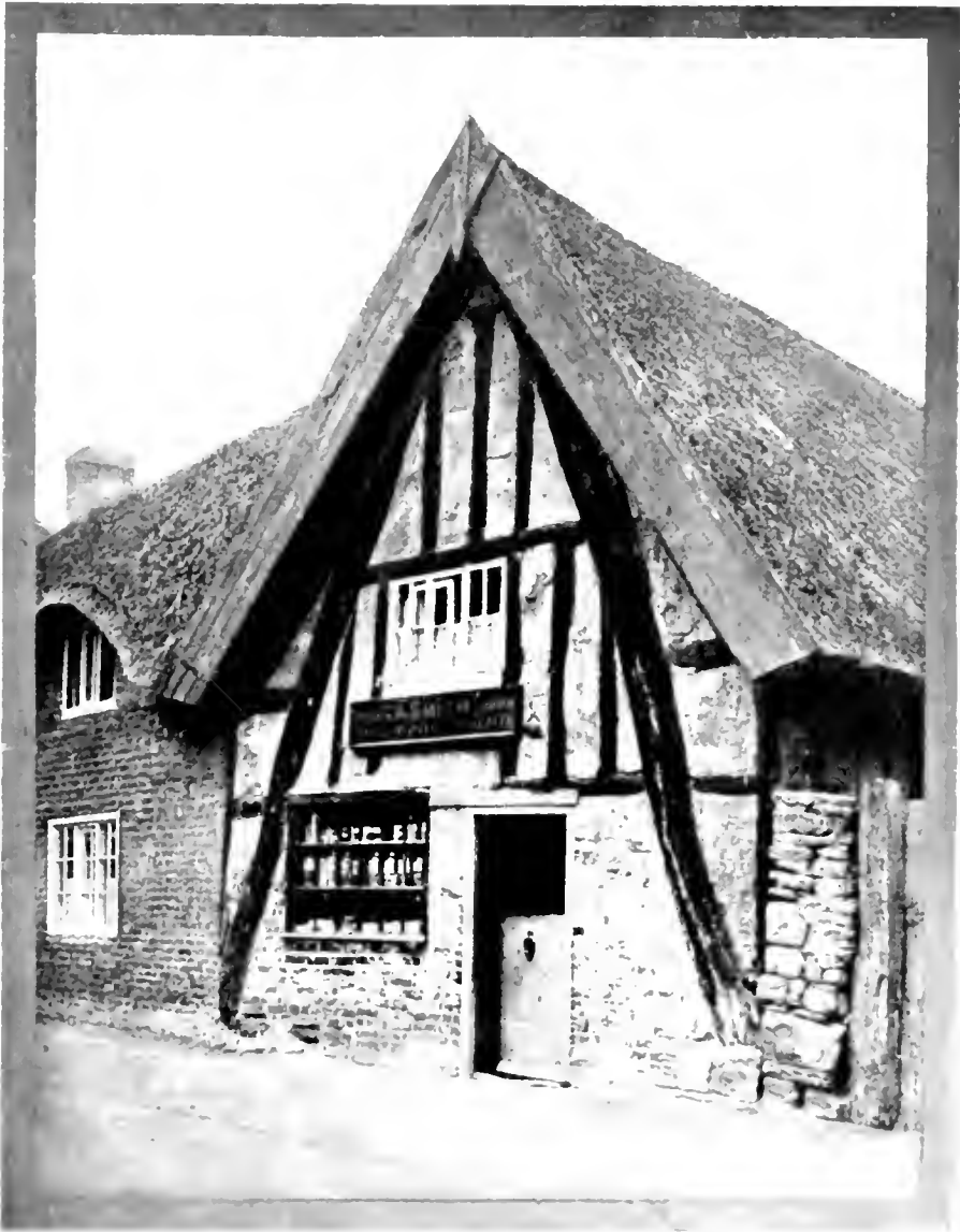
A cottage at Hetherington, Leicestershire, which is particularly interesting as a survival of the earliest form of timber construction
