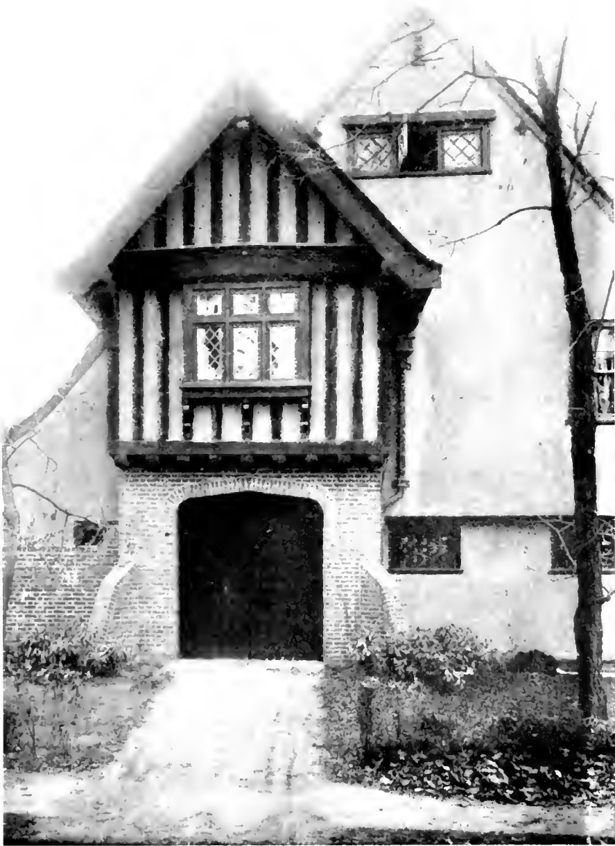
The plan of the half-timber house, by reason of its pliability, may provide, as here, for incorporating the garage into one end of the building
