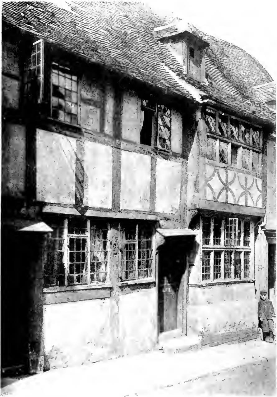
One of the essentials of success in half timber work is the grouping of windows rather than leaving them as isolated units
