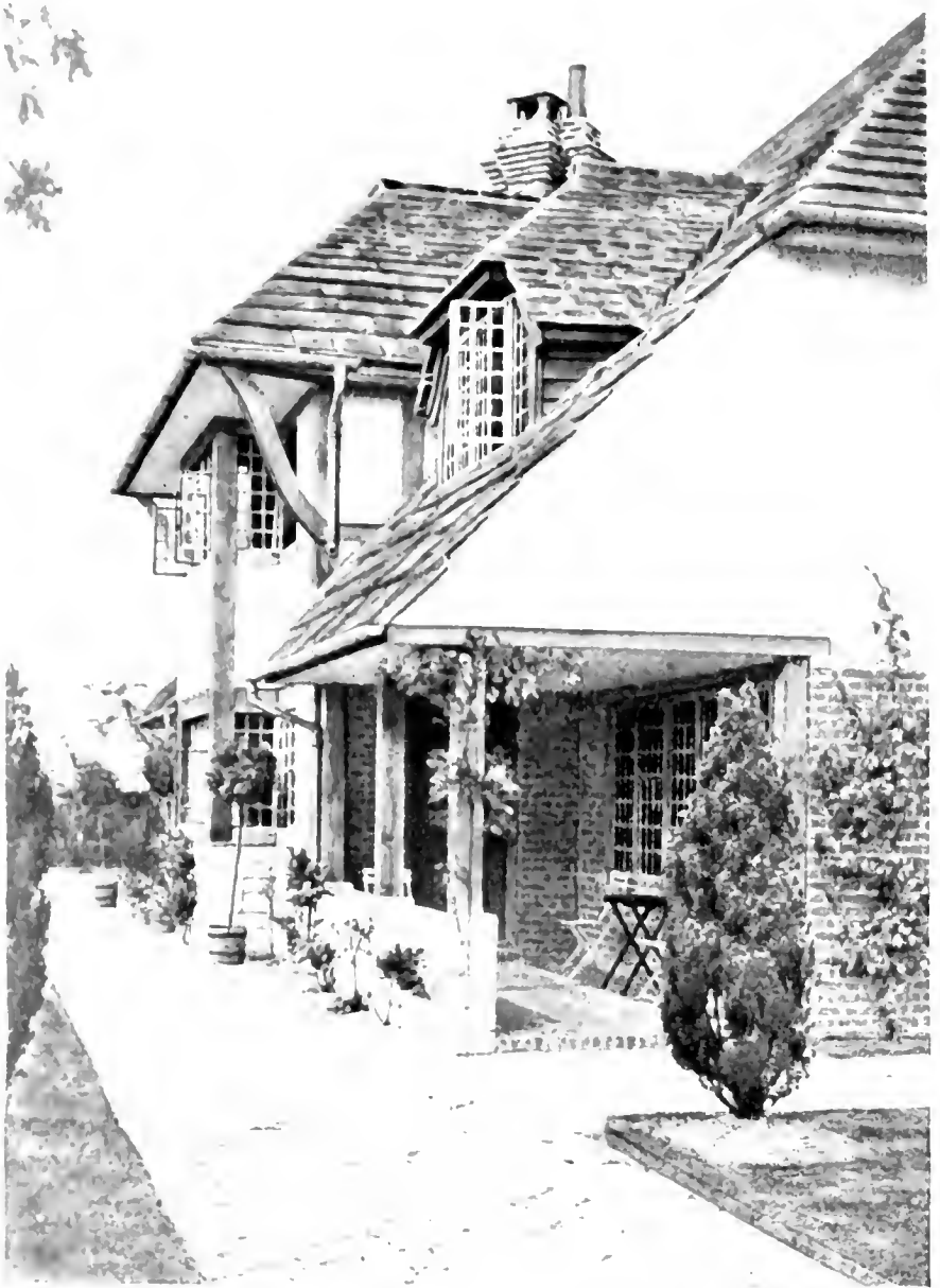
Half-timber work of the present day is seen at its best in conjunction with other materials, where the contrasting pattern between the plaster and the wood work is kept very simple, or restricted to use for features of the building that need accent.
