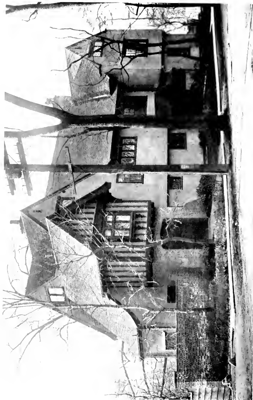
The garage is incorporated into the service end of the house, thereby incidentally avoiding the discomforts of a cold work-room and the freezing of water in the car's radiator
