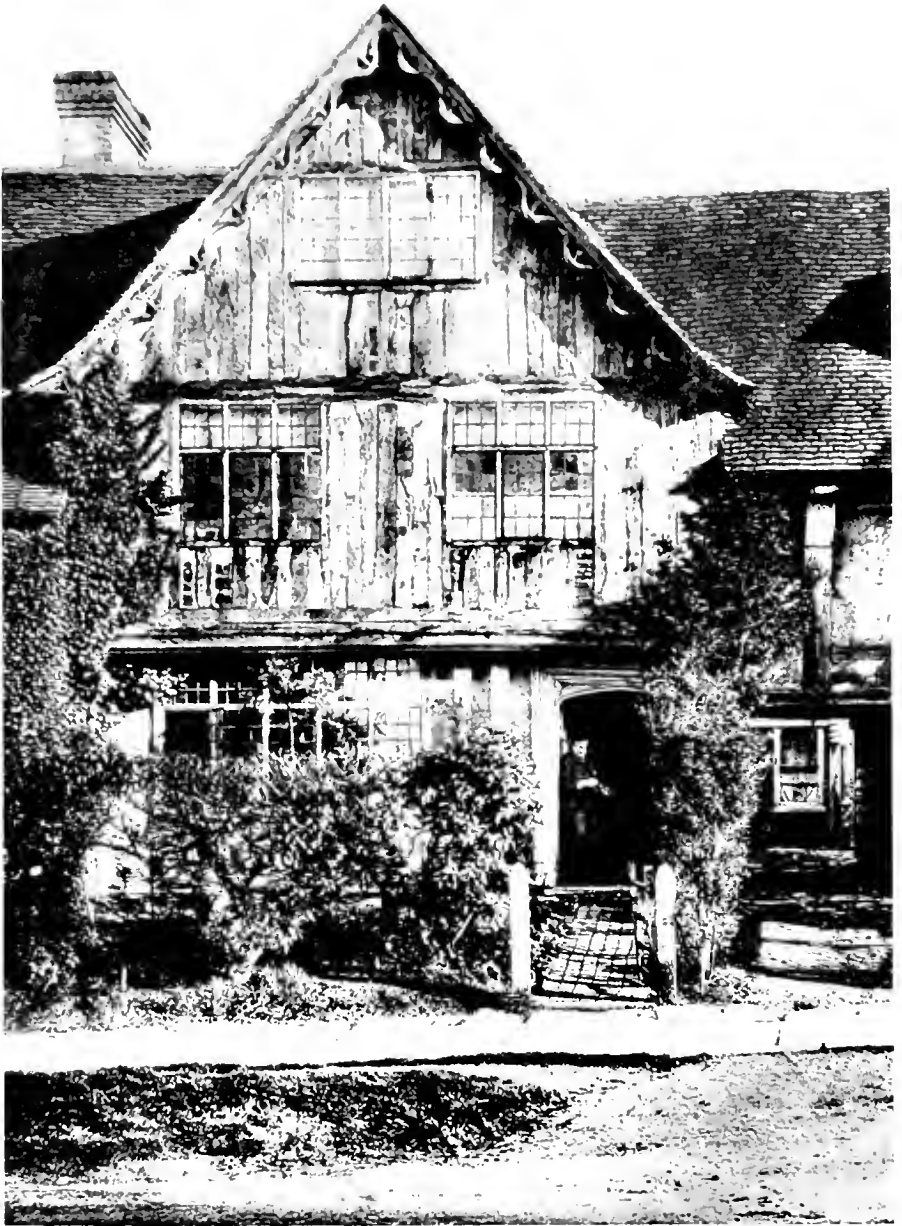
The sticks are vertical in the earlier work and rather close together, there being about as much plaster showing as wood
