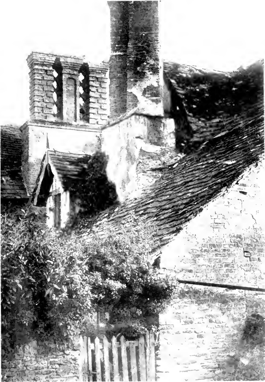
An admirable example of the charm of soft texture that resulted in the old work from the fact that it was not built with mathematical exactness
