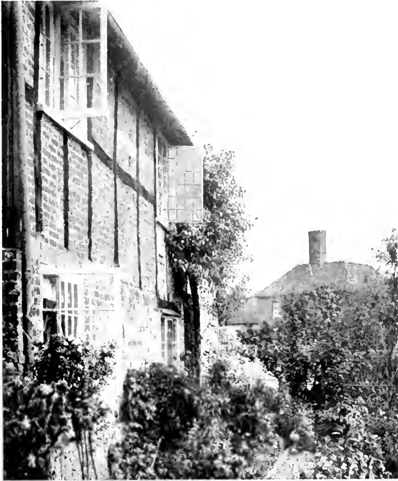
Casement windows and small panes both belong inseparably to the half-timber house
