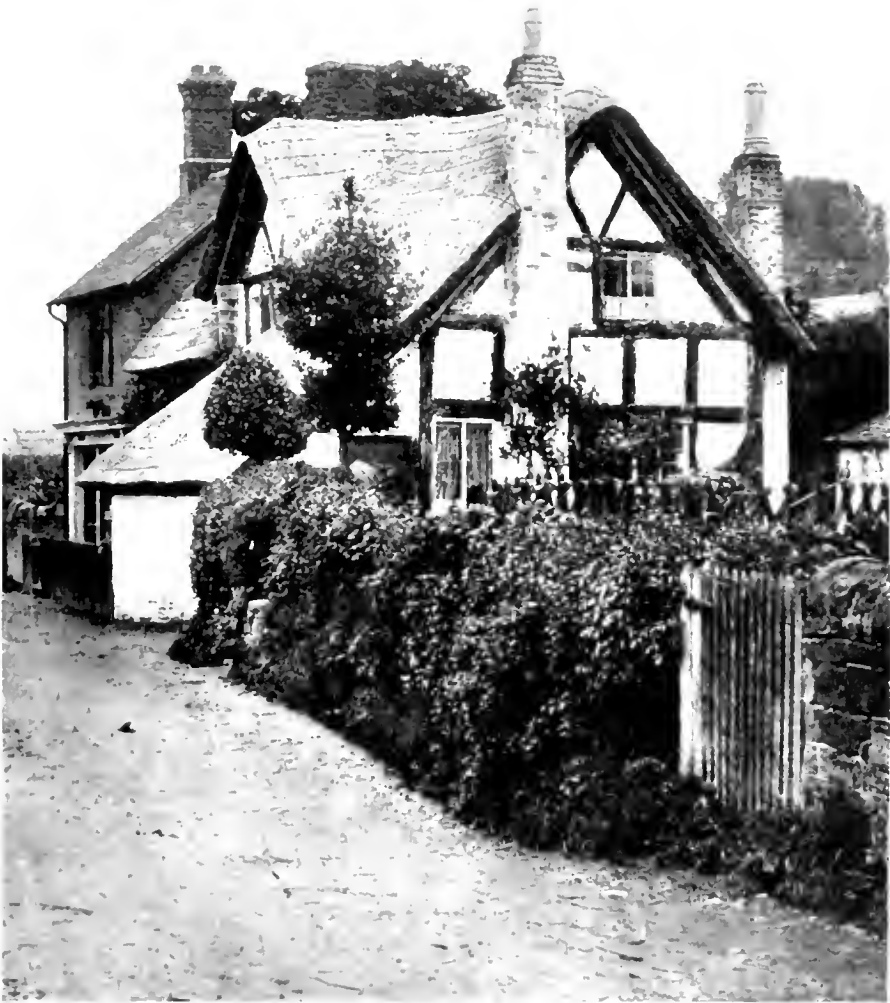
A wider spacing of the timbers marked the later work, after the builder had begun to realize the possibilities of this pliable form of construction
