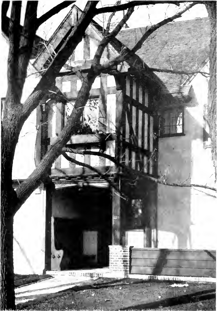
The timbering and other outside woodwork should be left rough and unpainted
