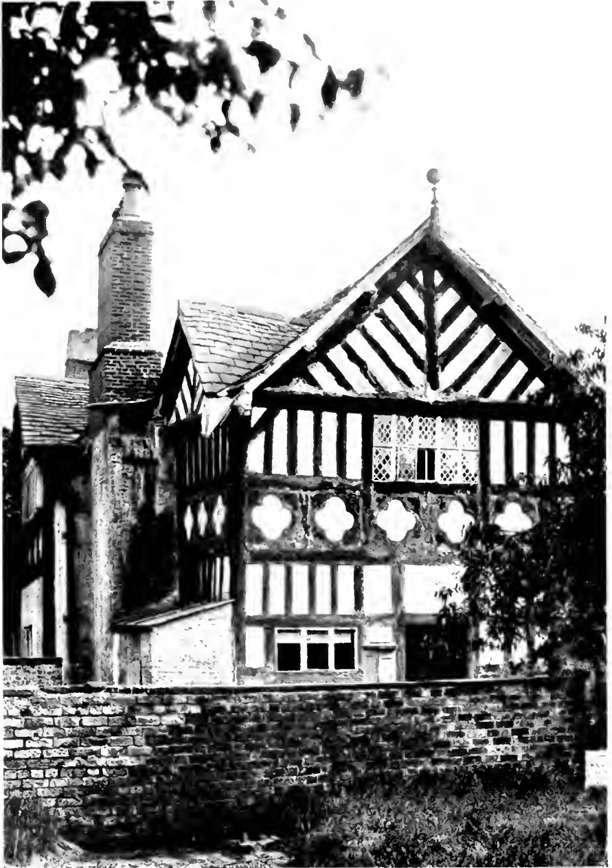
The builders soon broke away from the use of vertical timbers alone, introducing diverse and ingenious patterns such as the quatrefoil which is seen here
