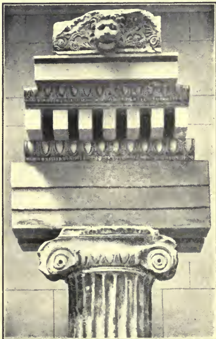
FIG. 97. — Ionic capital, architrave, and cornice, Priene. (Wiegand and Schrader, Priene , Fig. 71.)
