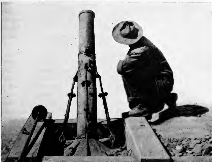
REAR VIEW OF MORTAR.
