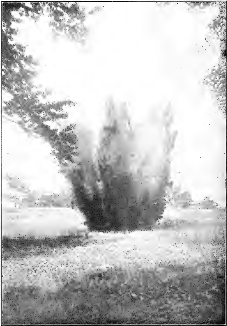
BLASTING A BOULDER
