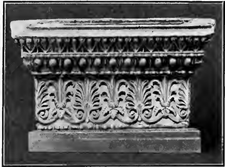
FIG. 99. — Attic Ionic anta capital, Erechtheum. (Photograph.)
