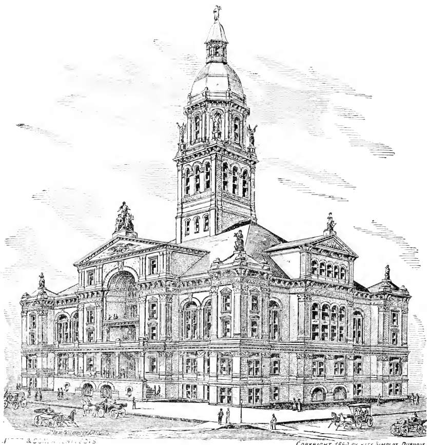
DUBUQUE COUNTY COURT HOUSE.
