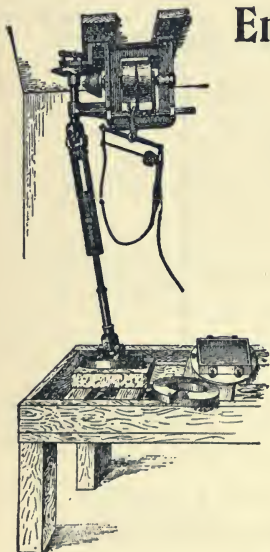
OVERHEAD LITHO. STONE GRINDING AND POLISHING MACHINE.
