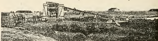
FIG. 162.—Dolberg's peat machine, with conveyer.
