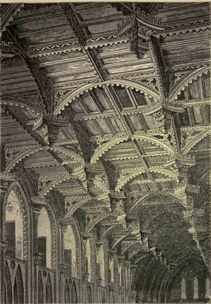
ST. DAVID'S CATHEDRAL. ROOF OF NAVE.
