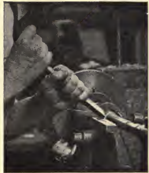
FIG. 8.—Turning iron with a graver.
