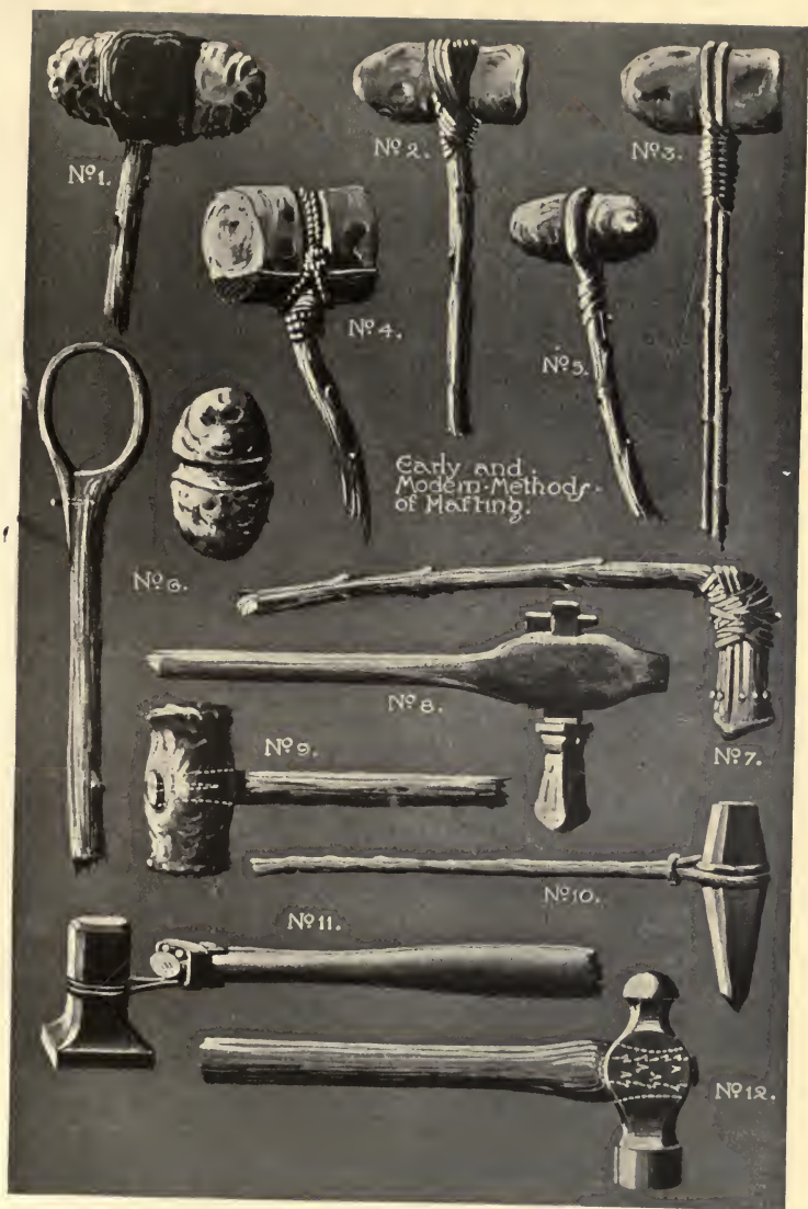
FIG. 5.—The evolution of the hammer.
