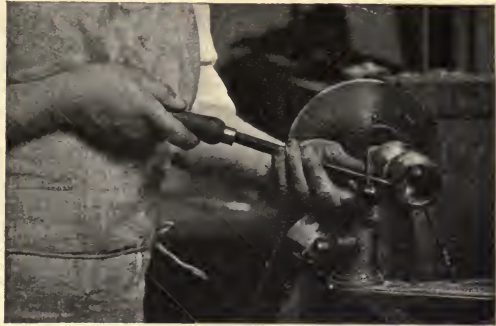
FIG. 7.—Turning brass with a ripper.
