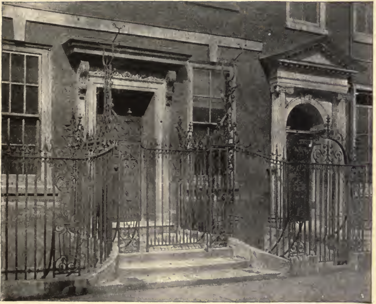
FIG. 2.—Ironwork at No. 44 Great Ormond Street, Bloomsbury (1708).
