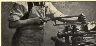
FIG. 17.—Method of holding a hack saw.
