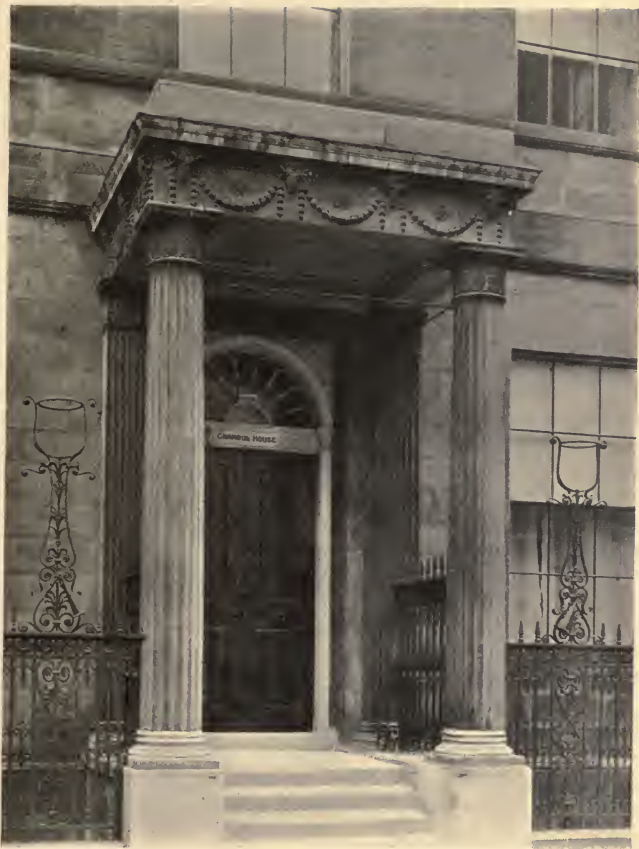
FIG. 1.—Portico and railings at Chandos House, Queen Anne Street, London. By R. and J. Adam.
