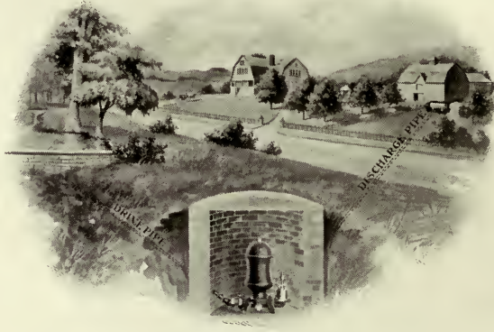
The Hydraulic Ram in Operation
