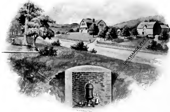
The Hydraulic Ram in Operation
