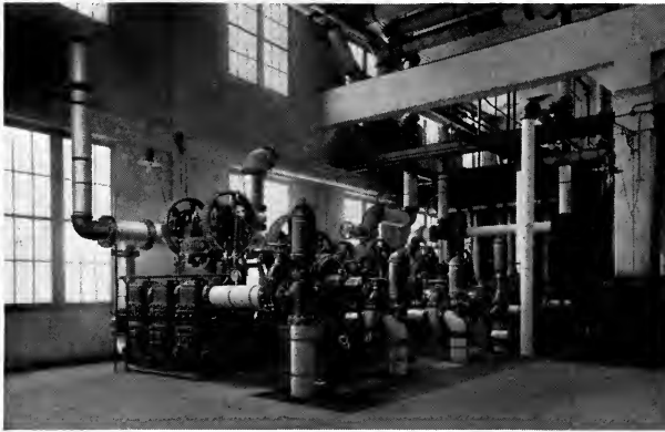
Installation of Deming Triplex Power Pumps in the plant of the Eastman Kodak Co., Rochester, New York
