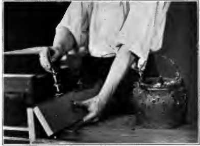
Fig. 260. Applying Glue for an Edge-to-Edge Joint.
