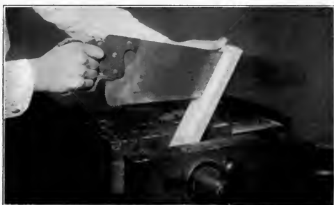
Fig. 89. Rip-sawing with Wood Held in Bench-Vise.
