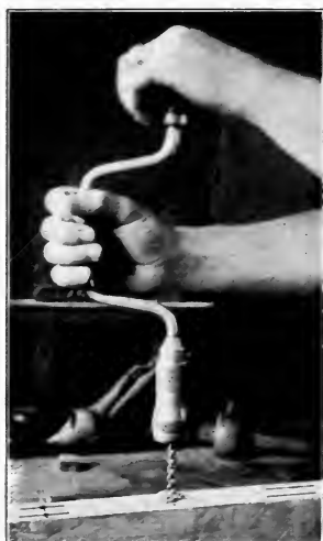
Fig. 263. Boring for Dowels in an Edge-to-Edge Joint.
