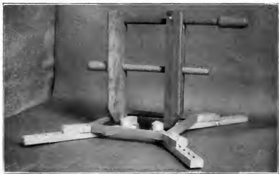
Fig. 254. Picture-Frame-Clamp.
