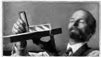
Fig. 105. Testing from Edge to Edge.
