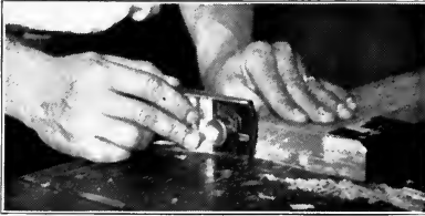
Fig. 109. Using the Block-Plane and Bench-Hook.
