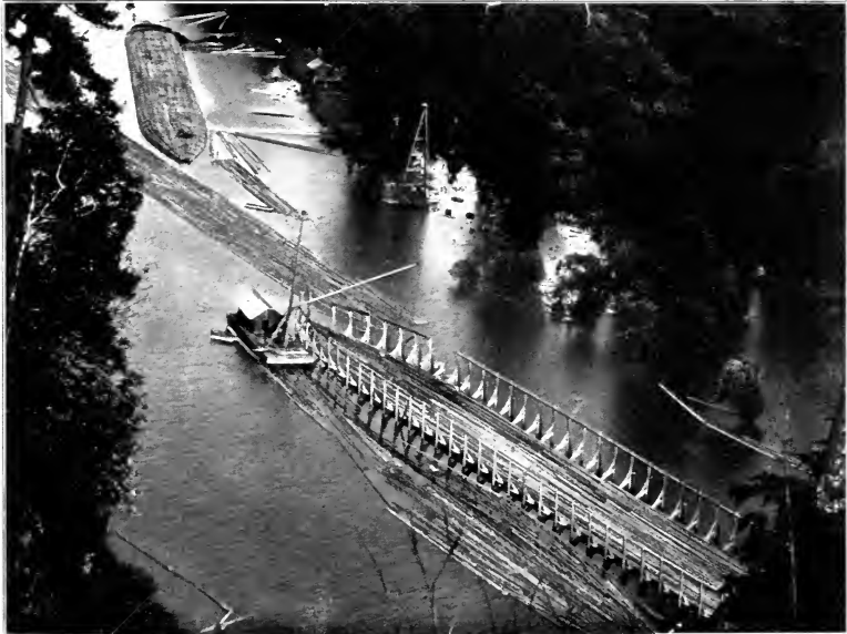
Fig. 30. Giant Raft. In the background is a completed raft; in the foreground a cradle in which a raft is being built.
