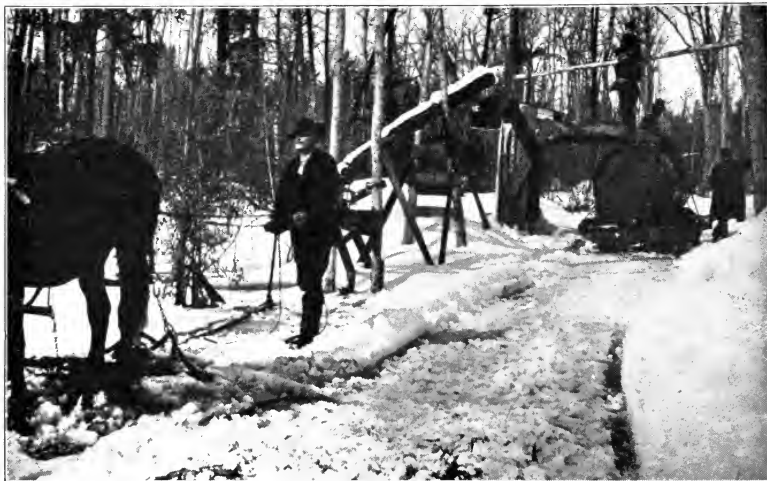
Fig. 10. Making an Ice Road by Flooding.
