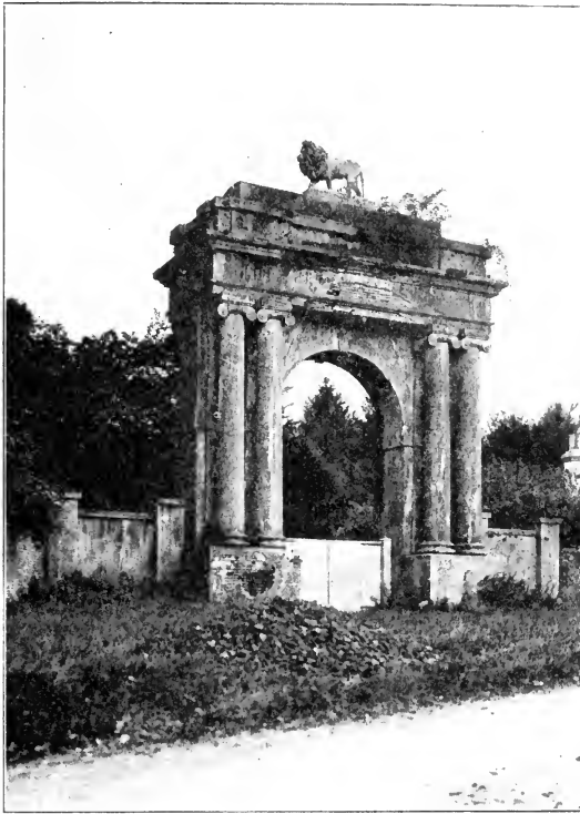
149.—CHARBOROUGH PARK ENTRANCE GATES.
