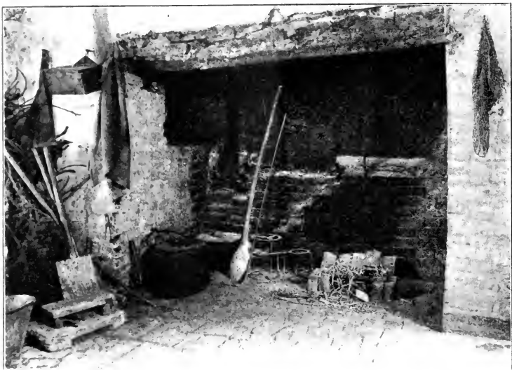
34.—INTERIOR OF THE BUCK'S HEAD INN, TROYTOWN.
