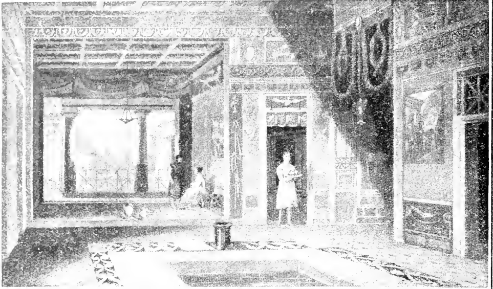
RESTORED INTERIOR OF THE "HOUSE OF THE TRAGIC POET"
