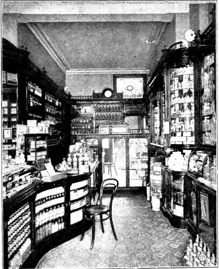
1. INTERIOR OF MODERN PHARMACY, SHOWING ADAPTATION OF VERY NARROW SHOP TO DRUG-SHOP FITTINGS
