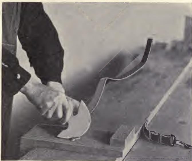
Fig. 10. Cutting the End of the Strap Square.
