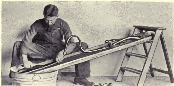
Fig. 42. Cleaning a Harness.
