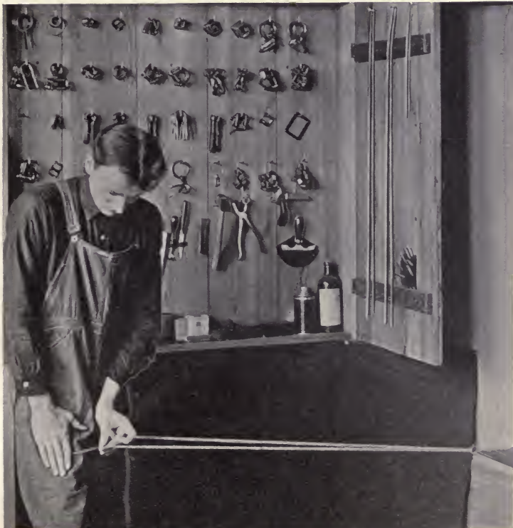
Fig. 6. Rolling the Thread on the Thigh to Twist It.
