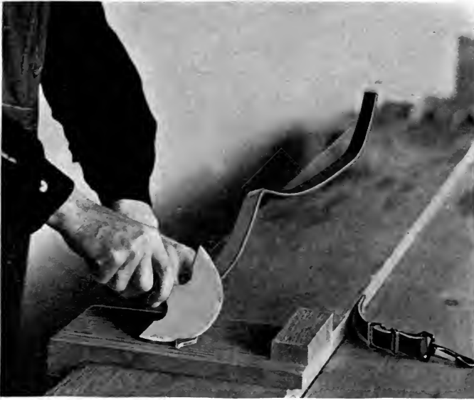
Fig. 10. Cutting the End of the Strap Square.
