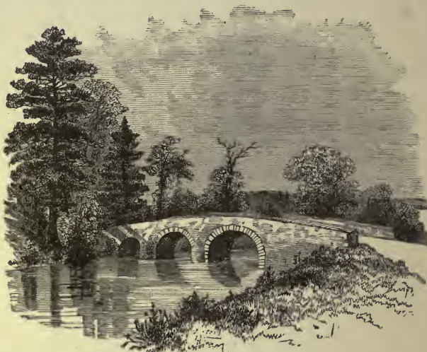
"BURNSIDE BRIDGE," ANTIETAM CREEK.
