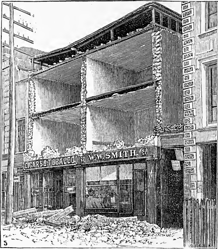
A RESULT OF THE EARTHQUAKE IN CHARLESTON, AUGUST 31, 1886.
