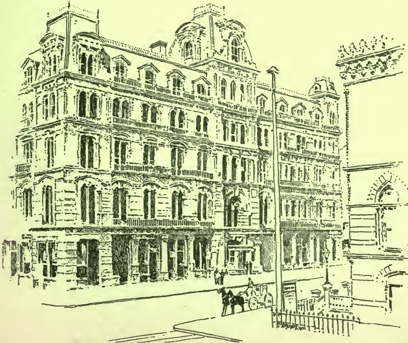
THE 23D STREET BRANCH, Y.M.C.A., NEW YORK CITY. TORN DOWN IN 1903.
