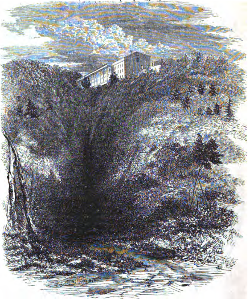
THE MOUNTAIN HOUSE.
