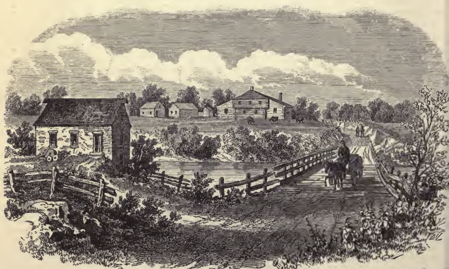
LA COLLE MILL AND BLOCK-HOUSE.
