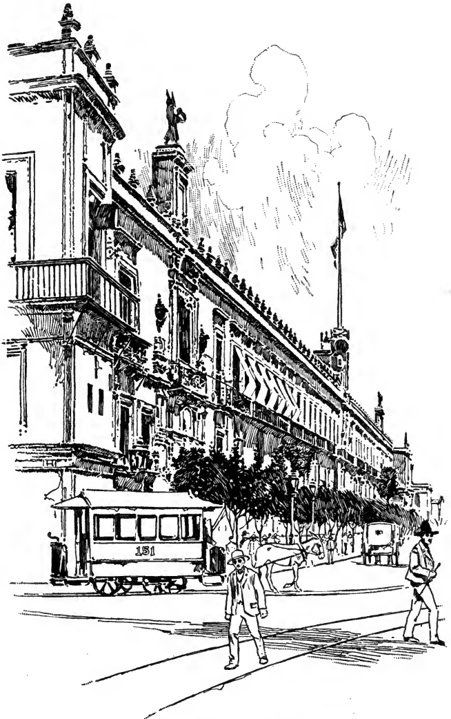
NATIONAL PALACE, CITY OF MEXICO.
