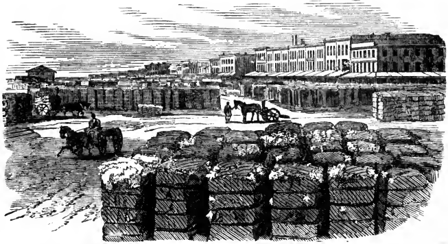
THE LEVEE AT NEW ORLEANS.
