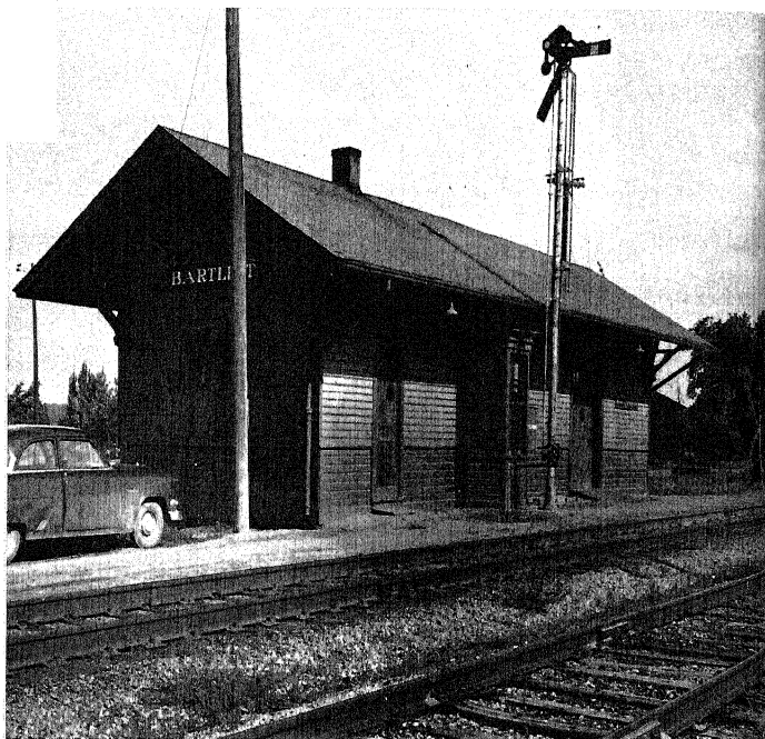
Burlington Lines photo Bartlett, Iowa, on the Burlington's "high iron" between Omaha and Kansas City. Bedwell issued train orders here and at other locals on this busy line along the Missouri River.
