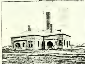
CITY WATER WORKS
