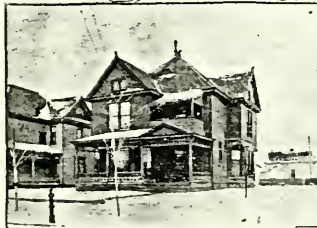
W. B. COOLEY'S RESIDENCE
