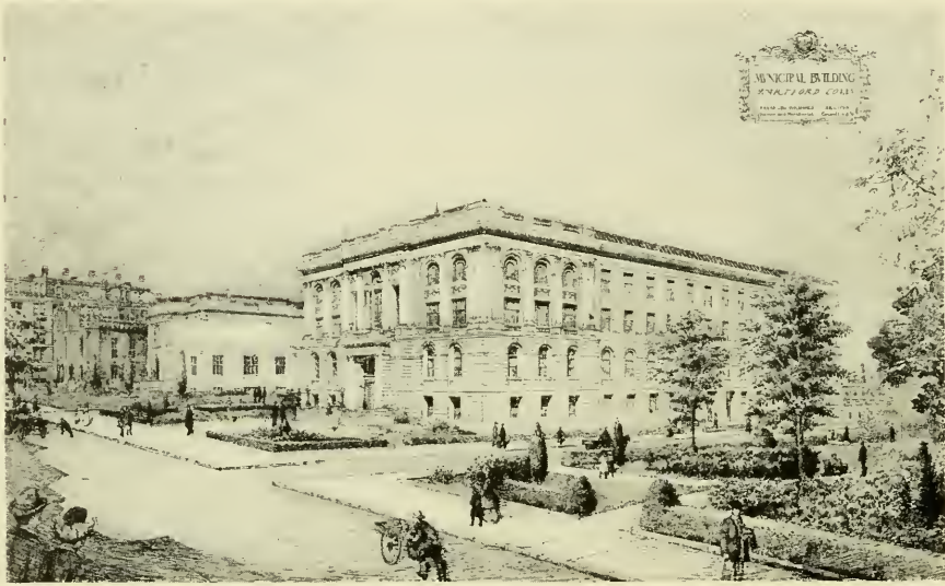
VIEW OF THE NEW MUNICIPAL BUILDING, HARTFORD The Norcross Bros. Co., General Contractors of New York, Boston, Washington, Providence, Worcester Davis & Brooks, Architects
