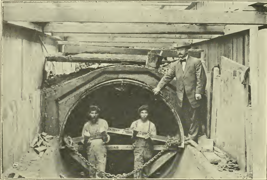
VIEW SHOWING THE O'CONNOR SYSTEM IN CONSTRUCTION.
