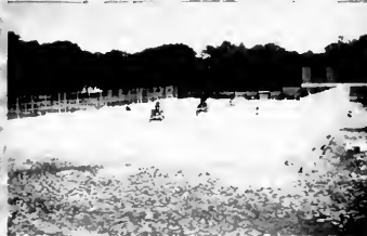
NEW TENNIS COURTS
