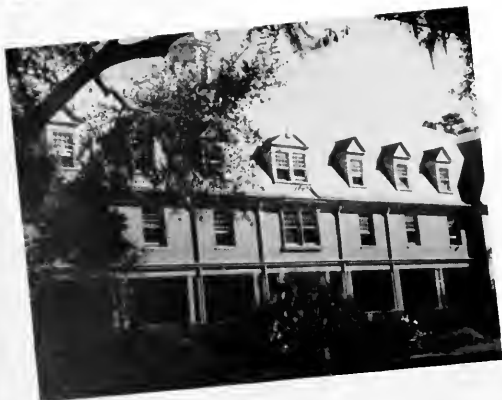
Conrad Hall Chaudin Hall
