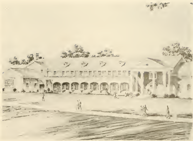
Student Union building—nearly completed.
