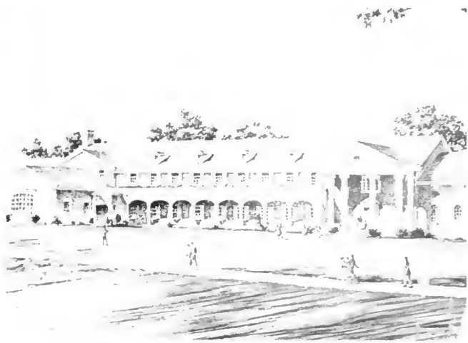
Student Union building—nearly completed.
